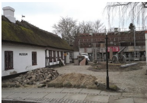
Mothsgården under renoveringen
